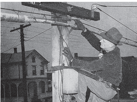
Lineman working with lead cables in photo from Bell Telephone Magazine.
