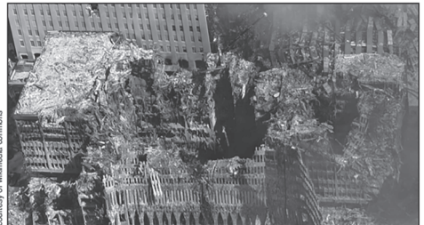
Verizon headquarters at 140 West Street in Manhattan, adjacent to the World Trade Center following the 9/11 attacks.
