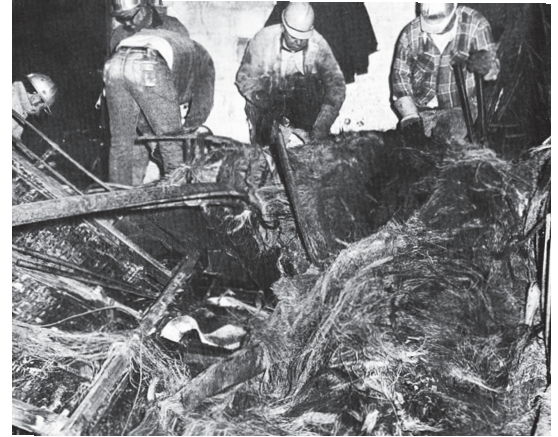
More than 700 FDNY members responded to the Telephone Company fire, which occurred on Feb. 27, 1975 at Second Avenue and 13th Street in Manhattan.
